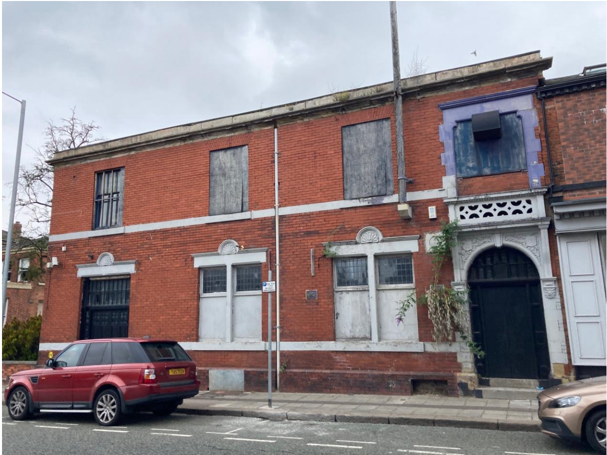
Photo 3: Building side elevation
